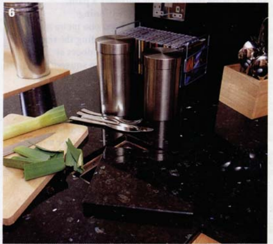
6 A section of granite in the preparation peninsula lifts out, so that food trimmings can be swept straight down into the waste chute
